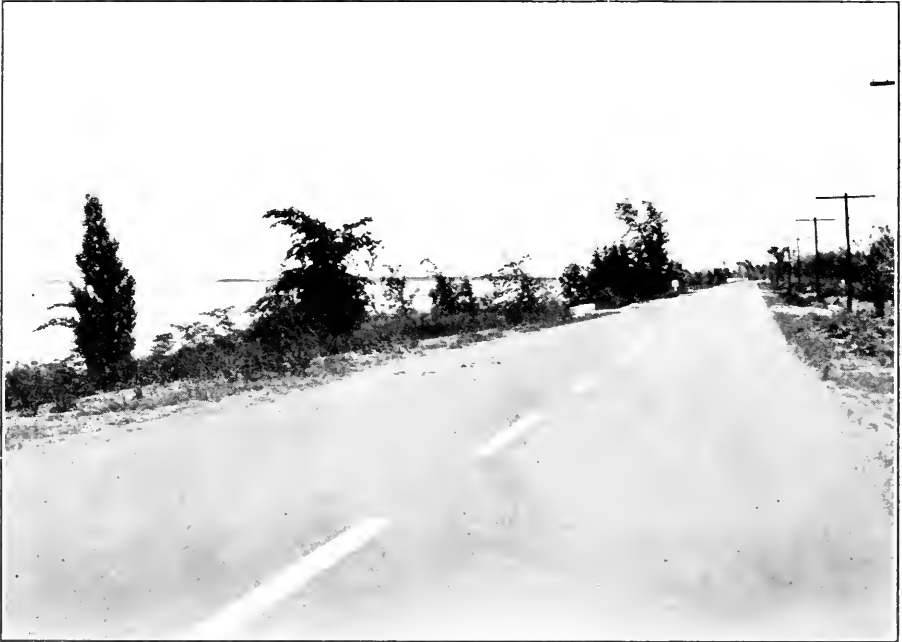
Mixed Macadam, Highway No. 26, West of Craigeleith.
